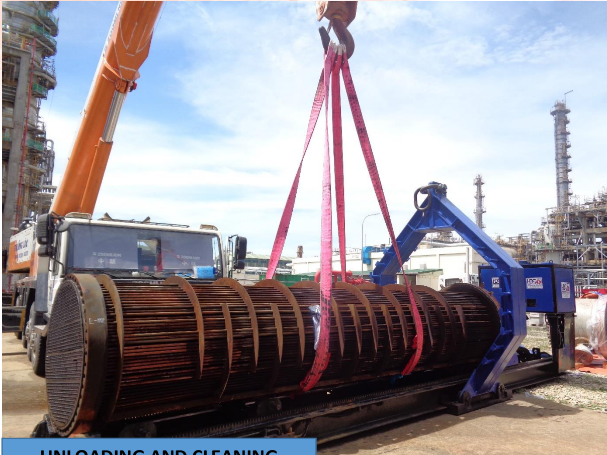
UNLOADING AND CLEANING EXCHANGER
