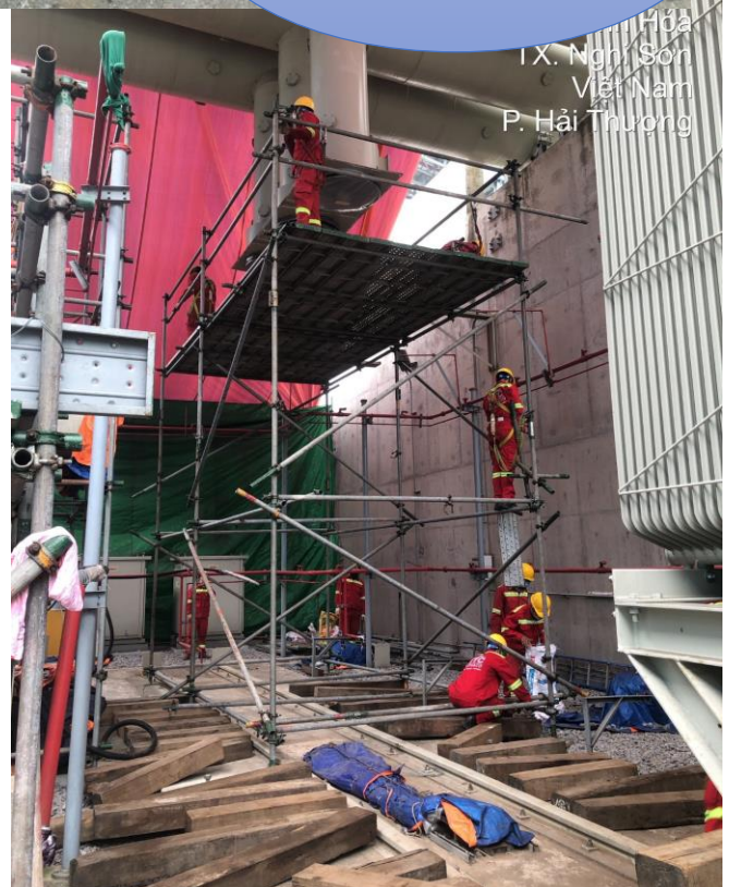
Unloading and dismantling transformer
