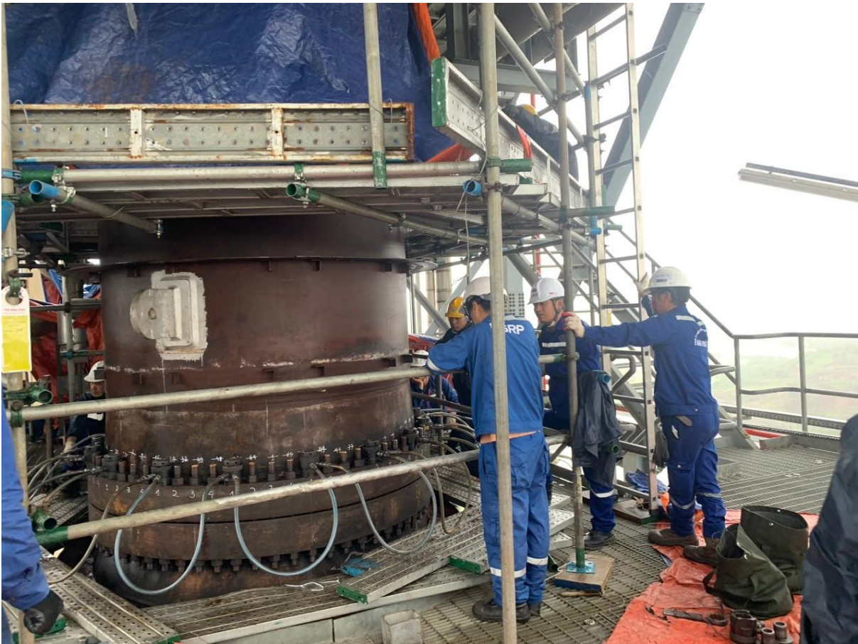
MECHANICAL WORK FOR TOWER
